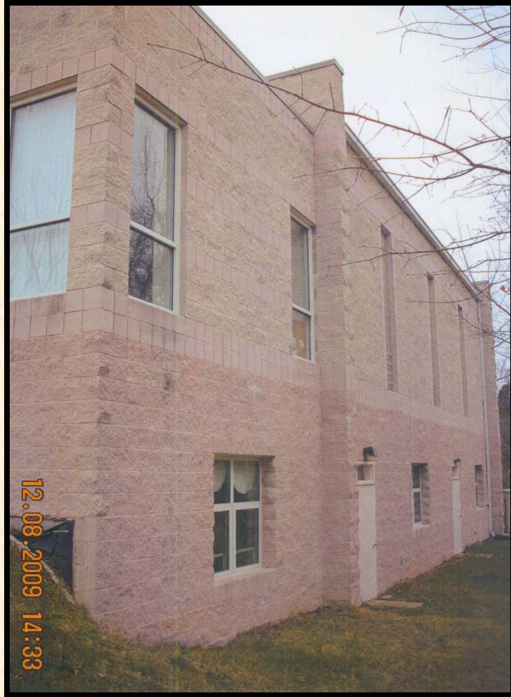
Less Visible South Side
