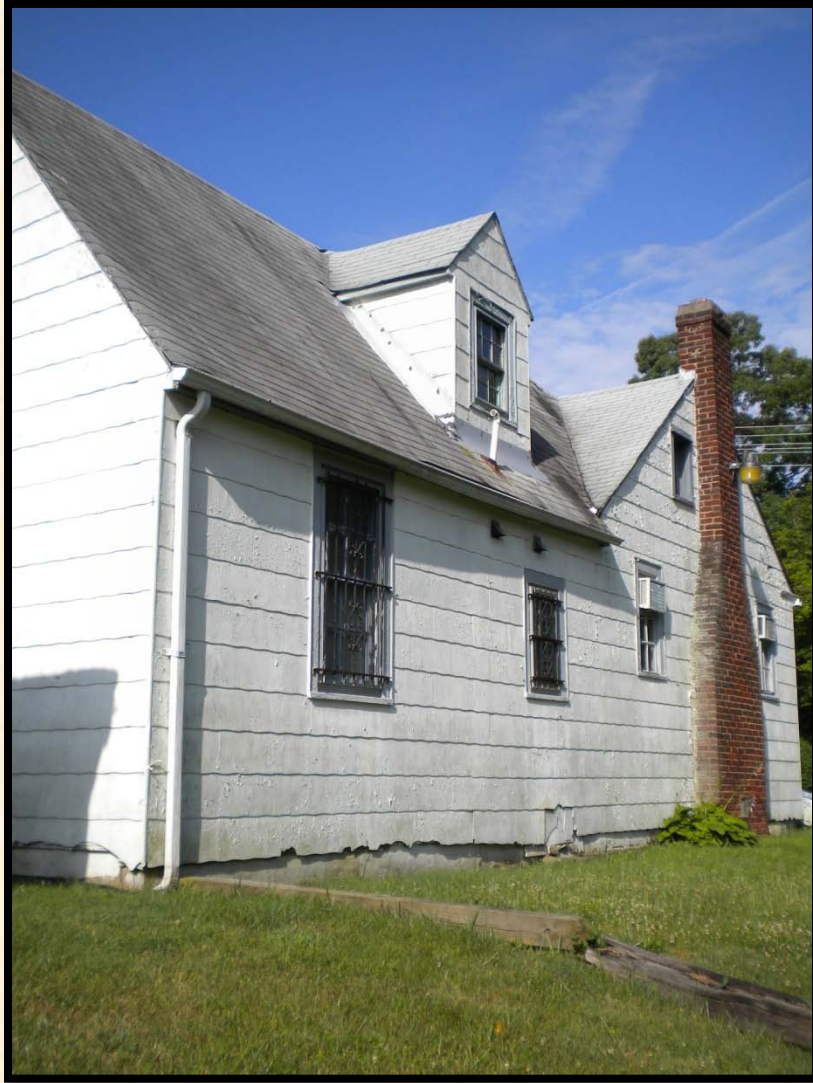
Existing building condition on the north (left) side
