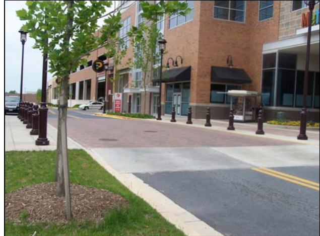
A raised crosswalk outside of the Metrorail station increasing the visibility of pedestrians while slowing down motor vehicles
