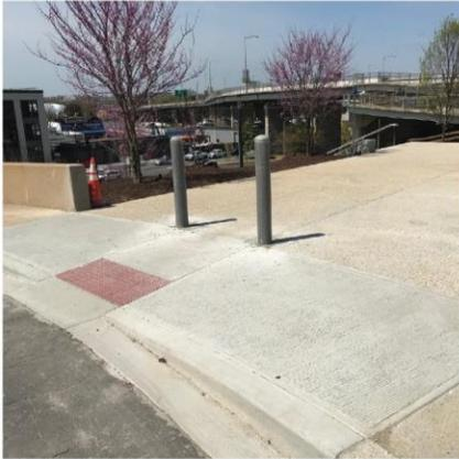
Curb Cut ADA Ramp with Bollards
