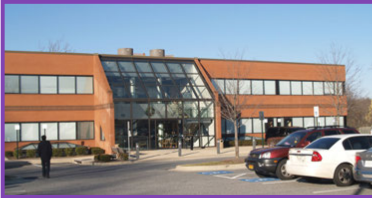
An office building just outside the Town of Upper Marlboro.
