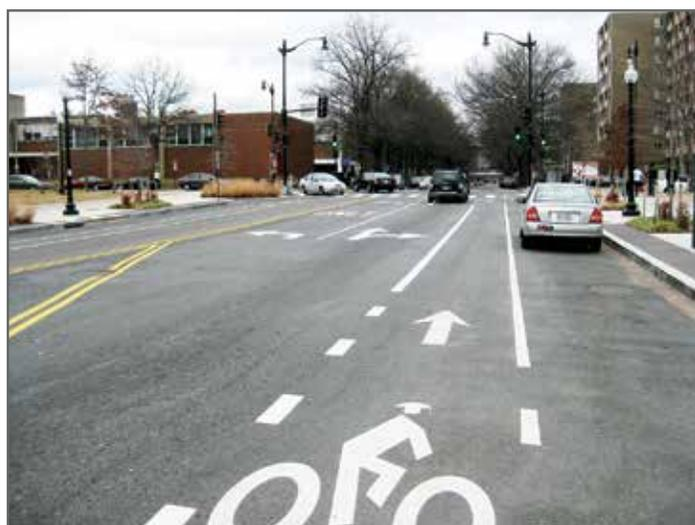
*This photo shows how lane markings can be used to accommodate a road narrowing while preserving the flexibility to transition back to a travel lane in the future.*
