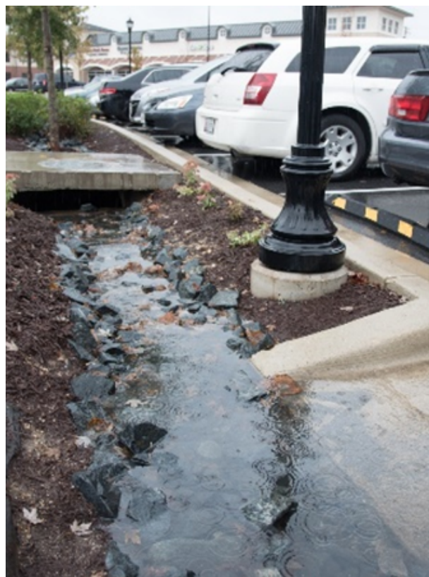
Figure 9. Functioning ESD stormwater feature at Bowie Town Center.
