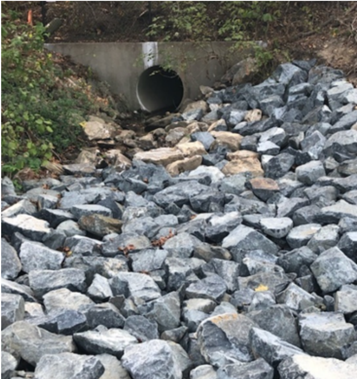
Figure 10. Strategic placing of riprap boulders to help prevent stream channel and streambank erosion. (Compare this photo with Figure 1.)
