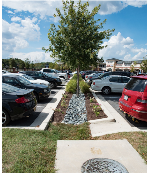
Figure 8. Part of the Bowie Town Center showing ESD technique to treat stormwater prior to its release to the storm drain system.
