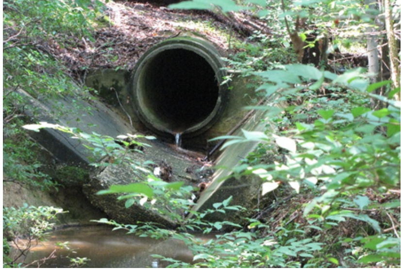
Figure 6. In parts of the plan area, stormwater from roadways and other impervious surfaces is channeled directly into receiving streams via concrete storm drains, severely impacting fragile ecosystems, as illustrated in Figure 7.
