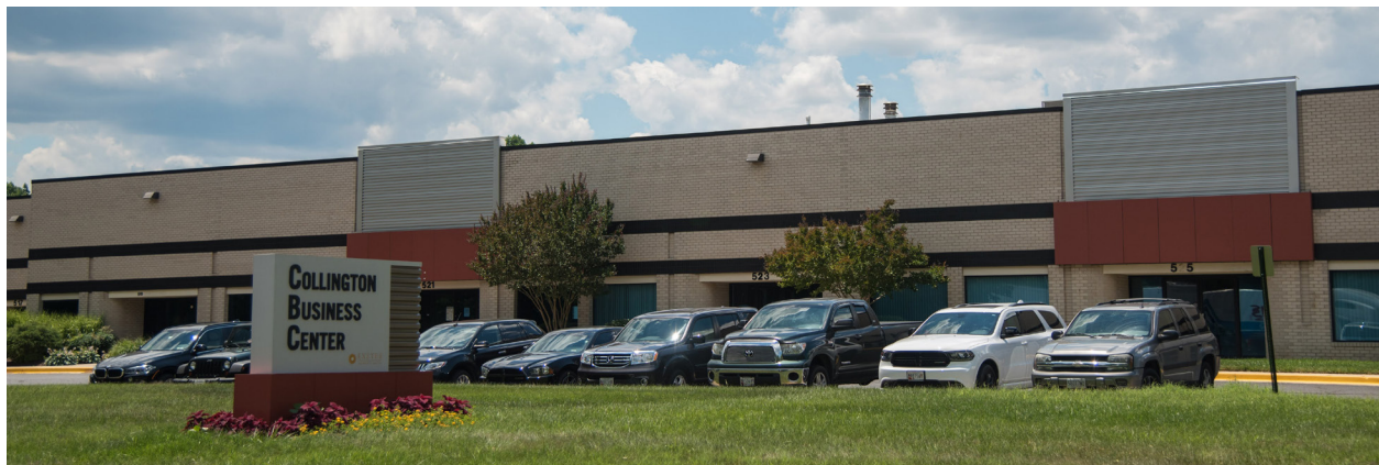
Collington Business Center within the Collington Local Employment Center
