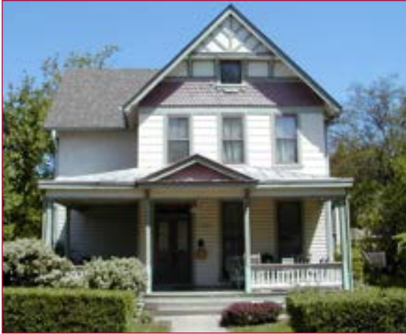
68-010-01 Welsh House 4200 Farragut Street Hyattsville
