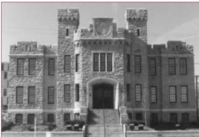
68-041-09 Hyattsville Armory (NR) 5340 Baltimore Avenue Hyattsville
