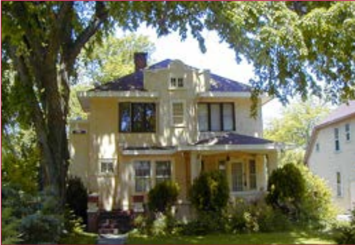
66-042-31 Holbrook House 4618 College Avenue College Park
