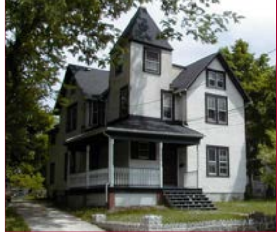
68-004-76 Wernek House 4606 Queensbury Road Riverdale Park
