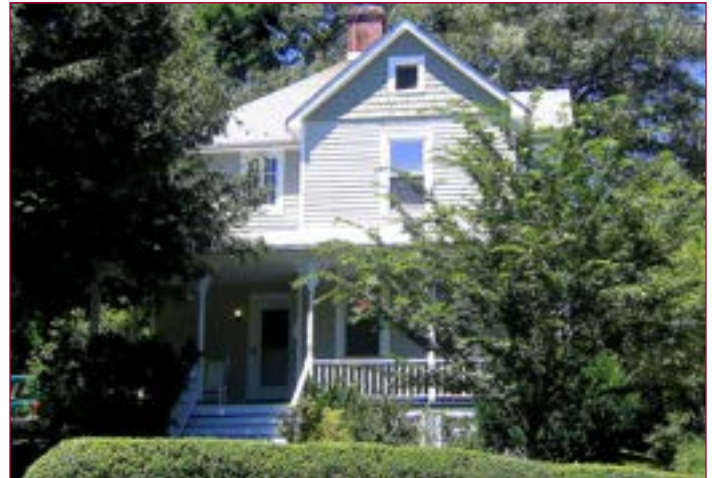
66-015 Buck-Singleton House 4908 Hollywood Road College Park
