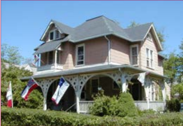
68-004-67 Read House 4722 Riverdale Road Riverdale Park
