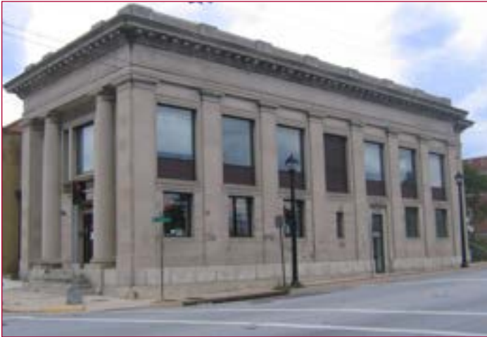
68-041-01 Professional Building 5200 Baltimore Avenue Hyattsville
