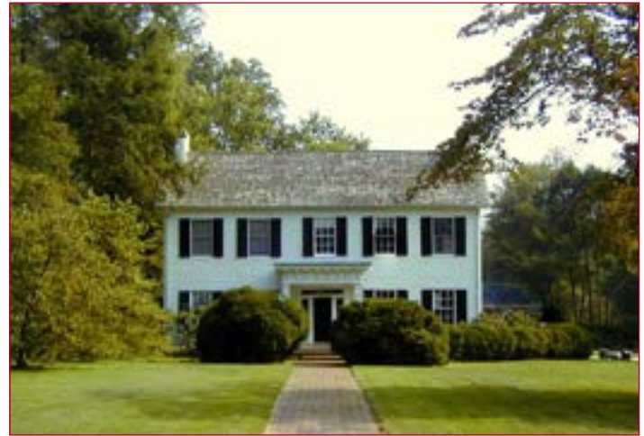
79-019-18 Digges-Sasscer House 14507 Elm Street Upper Marlboro
