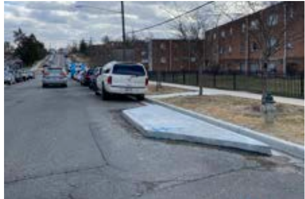
Recently installed curb extension on 15th Avenue.
