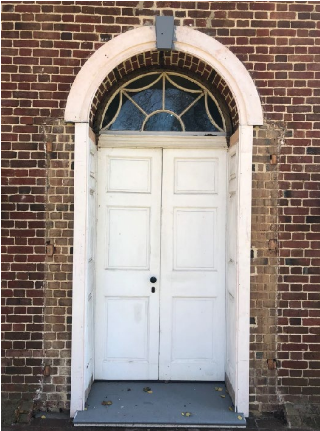
Masonry after completion of work.
