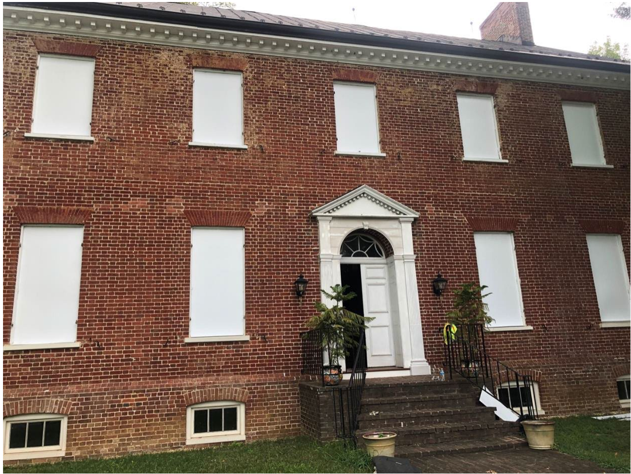
Front elevation before shutter restoration.
