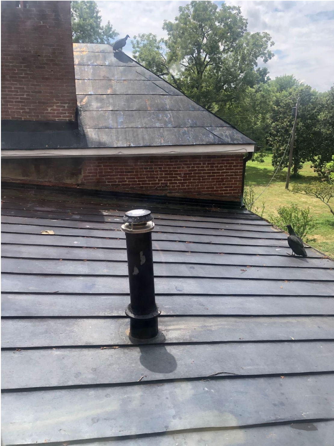
Kitchen and hyphen roof before completion of work.
