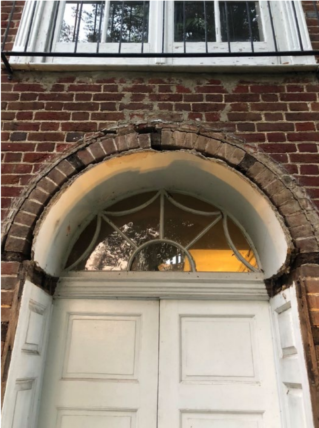
Masonry before completion of work.
