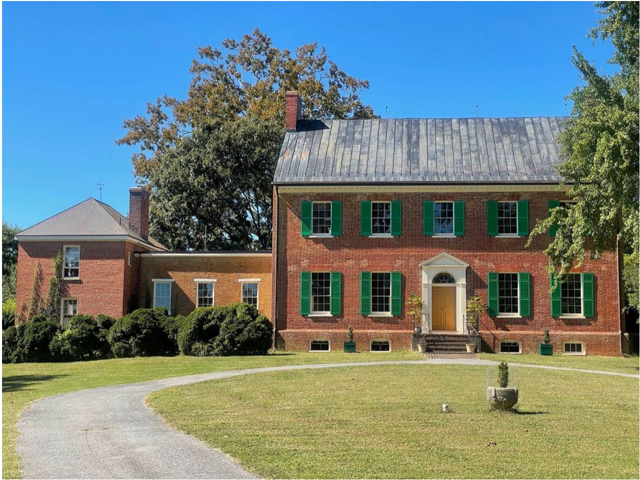
Front elevation after shutter restoration.
