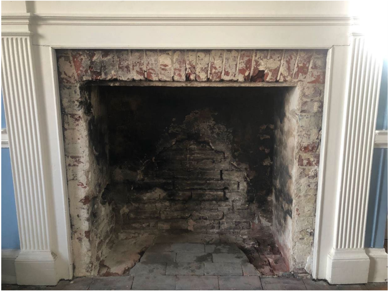
Fireplace before completion of work.
