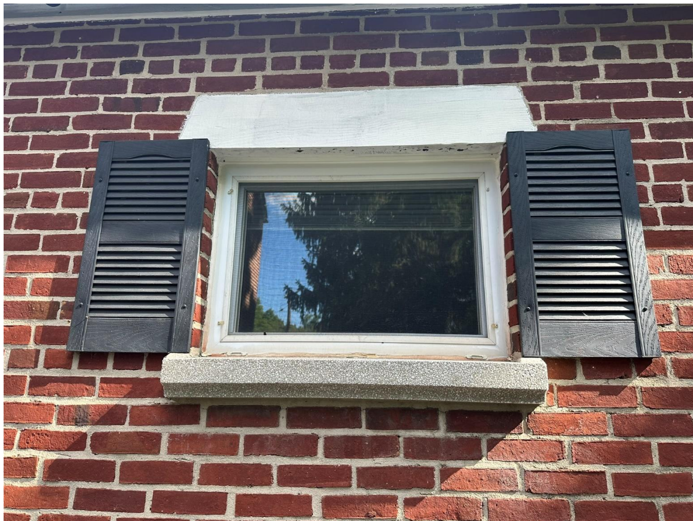
Detail, south elevation of garage showing a typical window with wood lintel and concrete aggregate sill, June 24, 2024.
