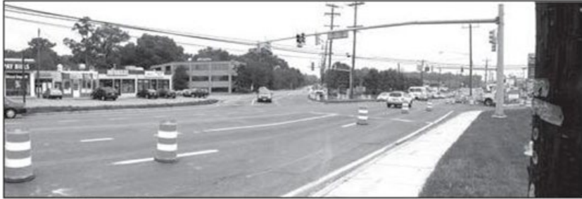
Rhode Island Ave. at US 1—Existing
