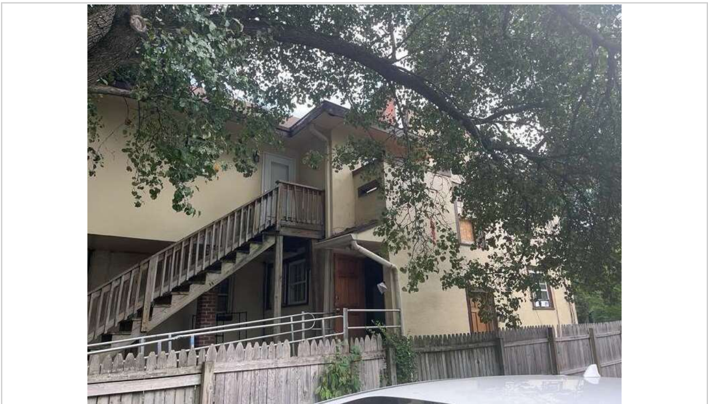
LT Side-Holbrook House, 4618 College Avenue-Windows/doors/Stucco and unique Trim Features-Alahambra Model Home- 7/30/24
