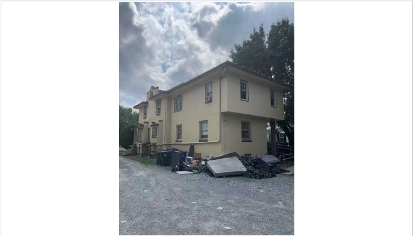
RT Side-Holbrook House, 4618 College Avenue-details targeted Windows/Stucco/unique Trim Features -Alahambra Model Home
