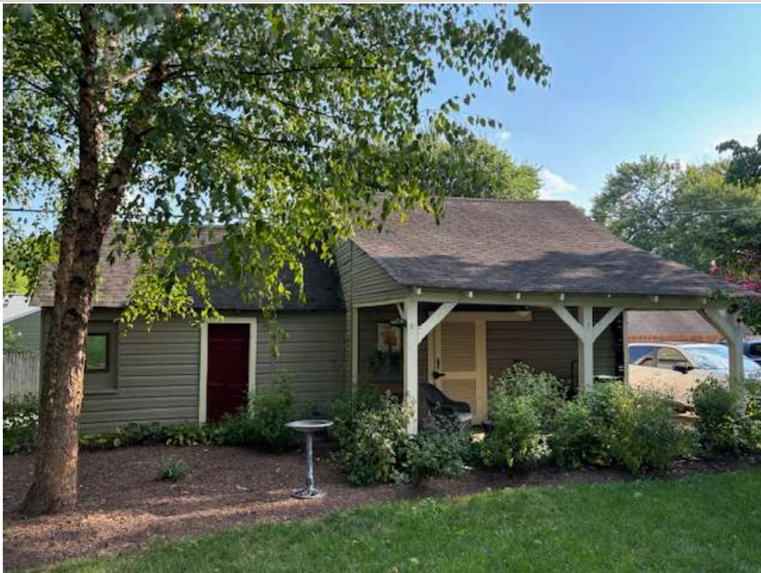
Garage - North side - Street view
