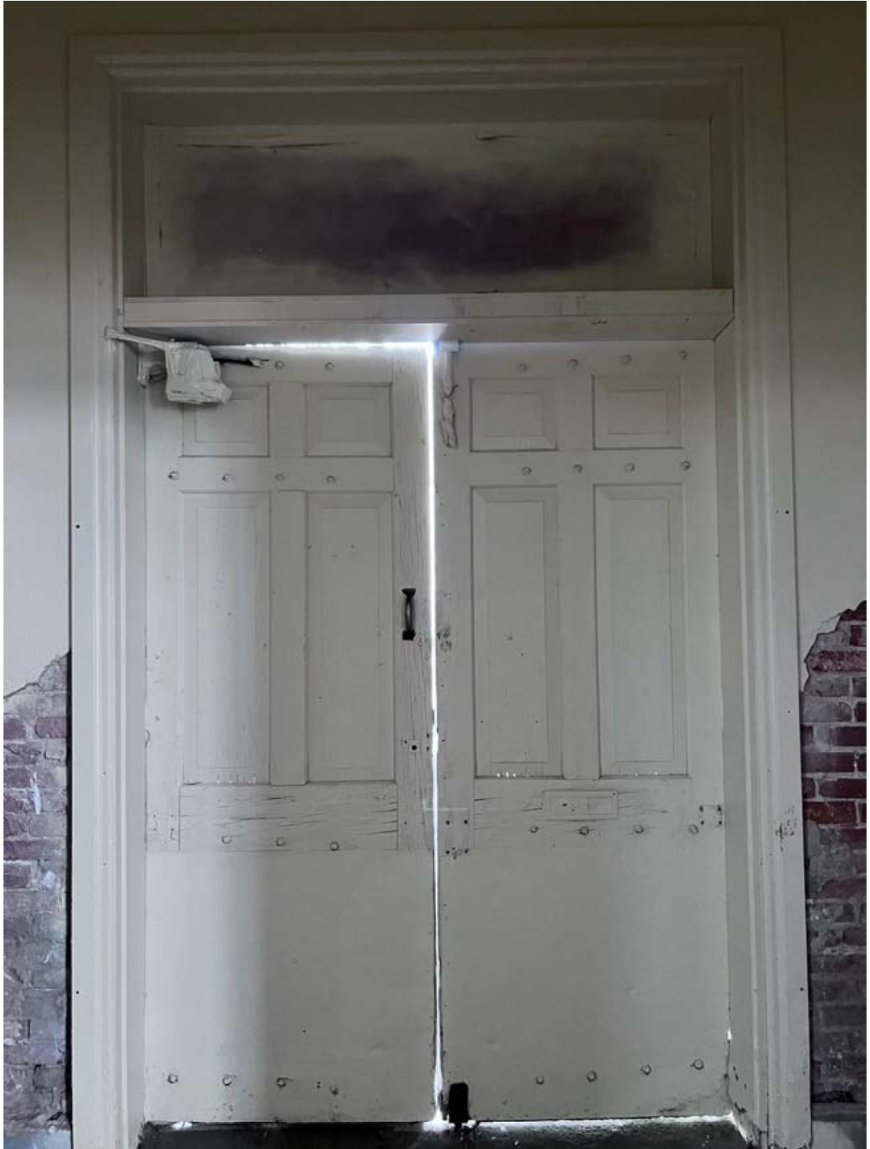
Front transom to be restored - June 2024
