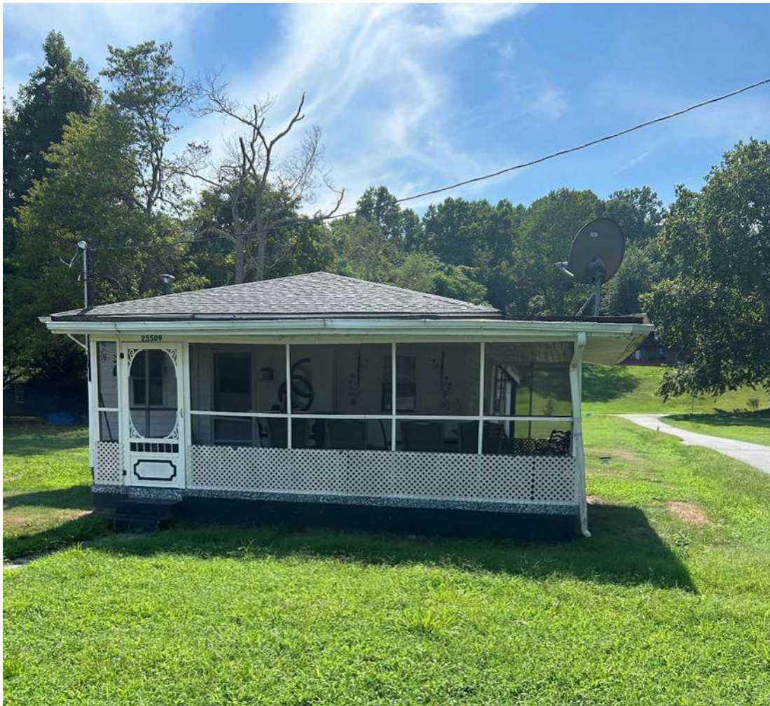
Figure 1- Front of house, east elevation facing the Patuxent River on the inland side of Patuxent Blvd, at intersection of Hawthorne Trail, a contributing building, dating to around 1946-53
