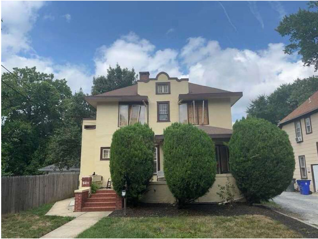
Front-Holbrook House, 4618 College Avenue-Windows/doors/Stucco and Unique Trim Features- Alhambra Model Home - 7/30/24
