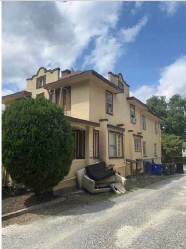
Holbrook House-details targeted Windows/Doors and Stucco and unique Trim Features Common to Alhambra Model Home
