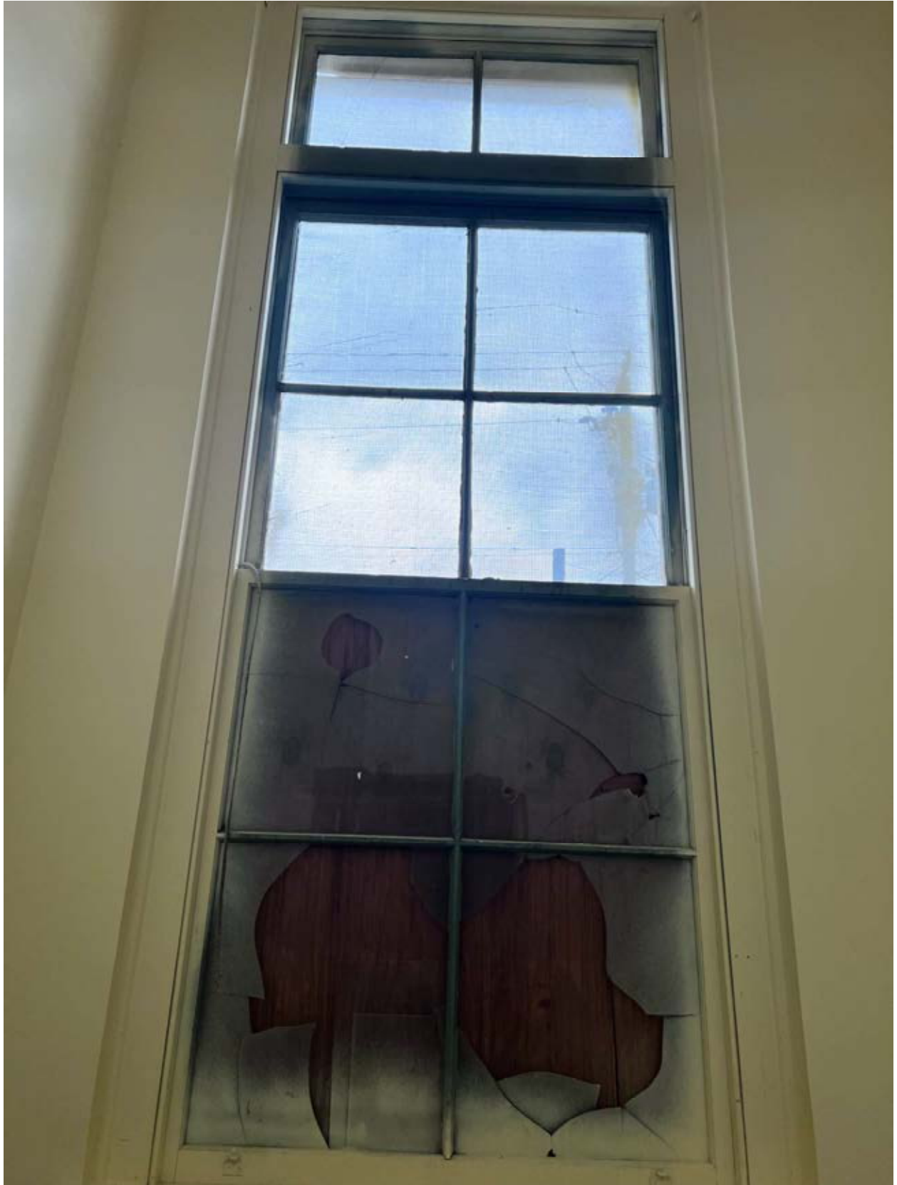
Existing front window to be restored - June 2024
