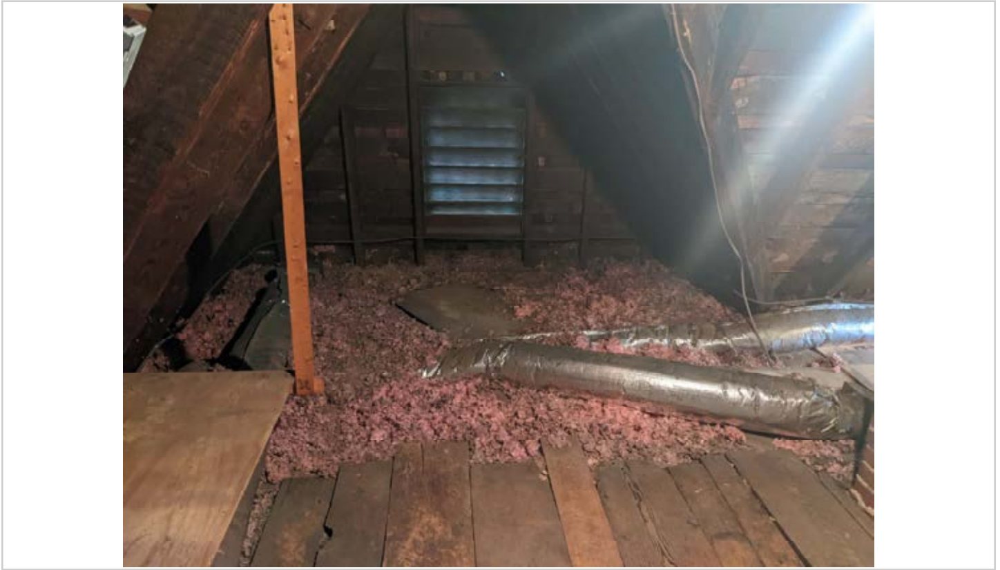
Loose fill fiberglass insulation in the attic (southeast), which will be augmented by air sealing and new fiberglass insulation. (8/9/2024)
