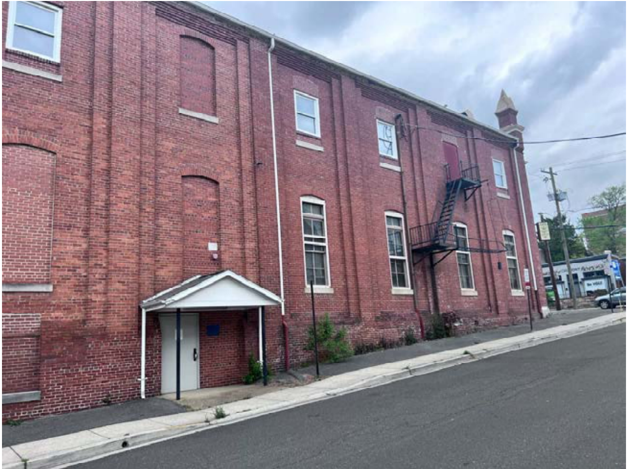
East elevation of subject property. Where there are bricked in window openings or vinyl replacement windows, these will be replaced with historic reproduction windows per the attached scope of work for this grant request. - June 2024
