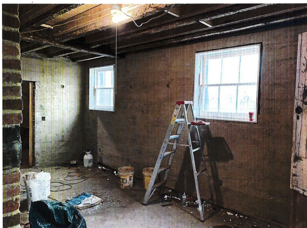
Figure 7: Kitchen after first coat of plaster work - December 2019
