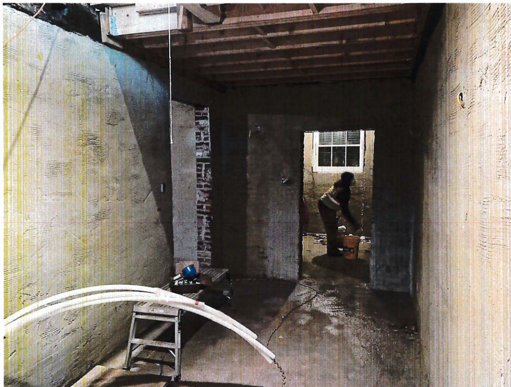
Figure 8: Downstairs hallway after first coat of plaster work - December 2019
