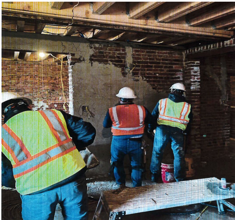
Figure 6: Lime plastering master bedroom - December 2019
