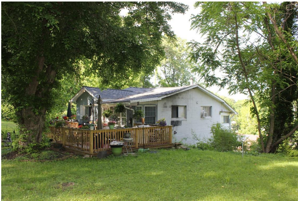
Photo 24 of 31 MD_PrinceGeorgesCounty_EagleHarborHD_0024.tif View of 23402 Wilson Drive, looking northeast
