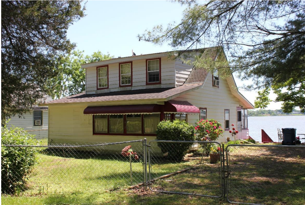
Photo 15 of 31 MD_PrinceGeorgesCounty_EagleHarborHD_0015.tif View of 23302 Patuxent Boulevard, looking northeast
