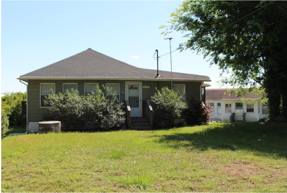
Photo 13 of 31 MD_PrinceGeorgesCounty_EagleHarborHD_0013.tif View of 18601 Trueman Point Road, looking east
