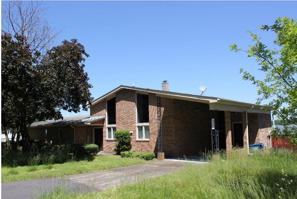
Photo 29 of 31 MD_PrinceGeorgesCounty_EagleHarborHD_0029.tif View of 23410 Patuxent Boulevard, looking northeast
