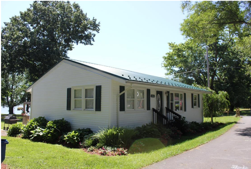
Photo 28 of 31 MD_PrinceGeorgesCounty_EagleHarborHD_0028.tif View of 18412 Juniper Trail, looking southeast
