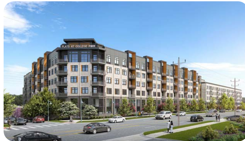
The Flats - under construction
