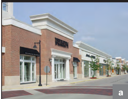
a) Buildings define the public sidewalk environment.
