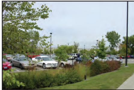
Typical example of bioretention area in a parking lot
