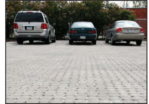
Typical example of permeable paving
